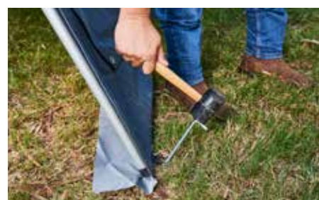
Pegging out the walls will help keep them quiet if it gets windy, as well as adding strength to the structure
